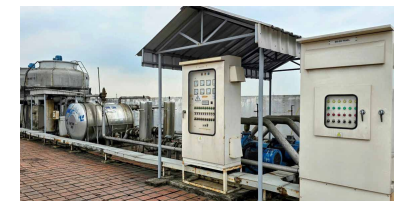
Energy-saving cooling tower system with inverter control
