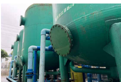
Final filtration tanks
